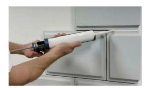
• The butt joints and mitre joints must be glued and grouted with the DOMOSTYL®HYBRID adhesive.
