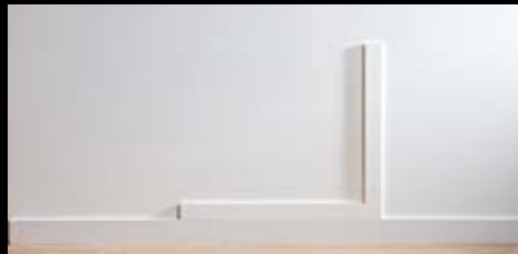
1. Run Multi Mould 4 across the bottom, at skirting board height.
