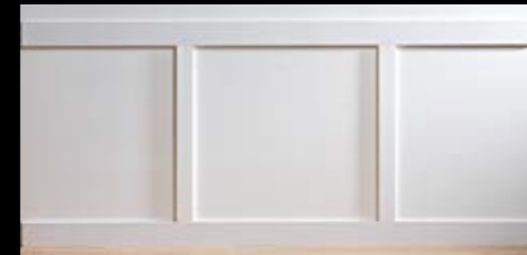
3. Add Multi Mould 4 across the top, at dado rail height.
