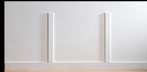
2. Add Multi Mould 3 as uprights. Spacings to your specification.
